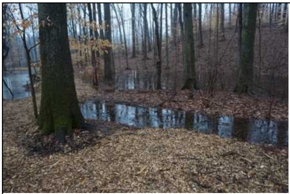
Figure 14. Depression shown in Figure 12 remains post construction. Hydrology was slightly altered due to the haul road that remained on site to serve as a footpath, but the depression continues to receive seepage from the slope and drain into the stream through the sand and woodchip filter.
