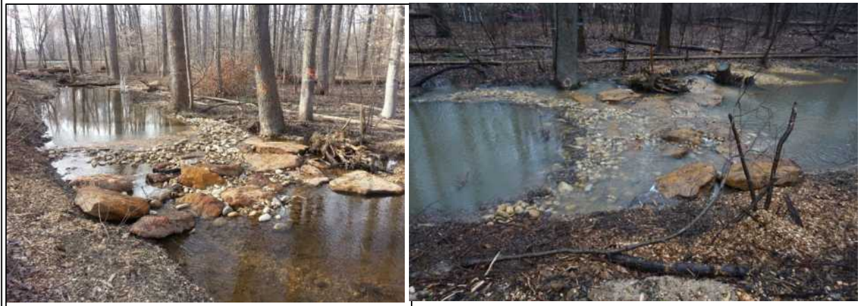
Figure 33. Riffle-weir constructed with weir boulders. From downstream to upstream (right side of photos to left), features are pool, river rock apron (submerged), footer boulder (exposed during baseflow conditions on left photo) anchoring the weir boulders that are controlling grade, riffle and pool. Note that the weir boulders are not stacked on top of footer boulders.
