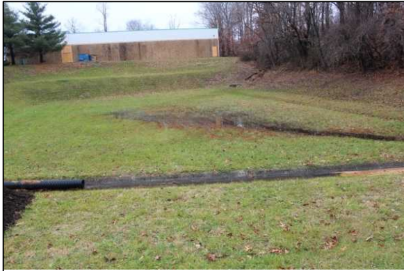
Figure 5. Example of a dry pond retrofit that created sand and woodchip berms and filter beds to increase time of stormwater detention and decrease volume and velocity entering the stream immediately below. This was a fill project.
