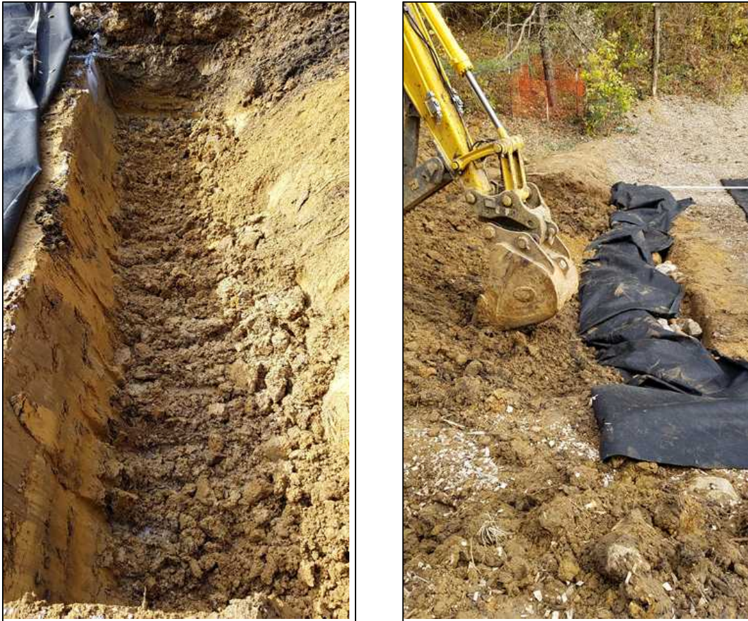
Figure 10. Smooth bucket creates smears (left vertical side of left photo) impeding subsurface flow; whereas toothed bucket “fluffs” the soils (bottom and right vertical sides of excavated area in left photo, and right photo) and allow movement of water vertically and laterally.
