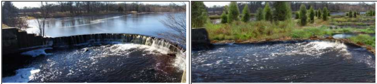
Figure 9. Example of dam removal and regenerative restoration of a stream with a 13-square mile drainage area. This was a fill project to improve water quality and fish passage.
