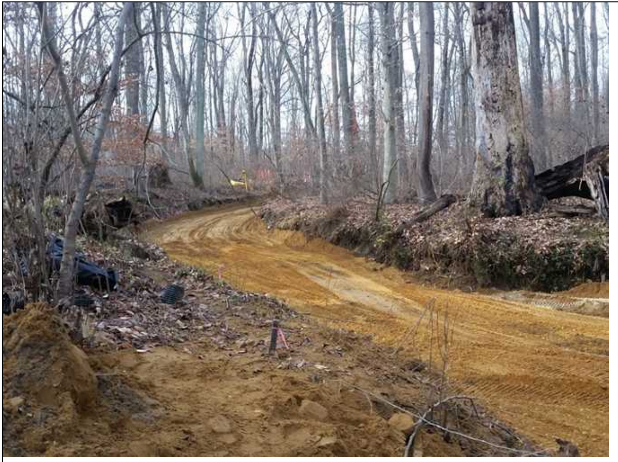
Figure 27. Woodchip and sand haul road constructed in stream to raise the stream bottom and to minimize impacts to riparian area.
