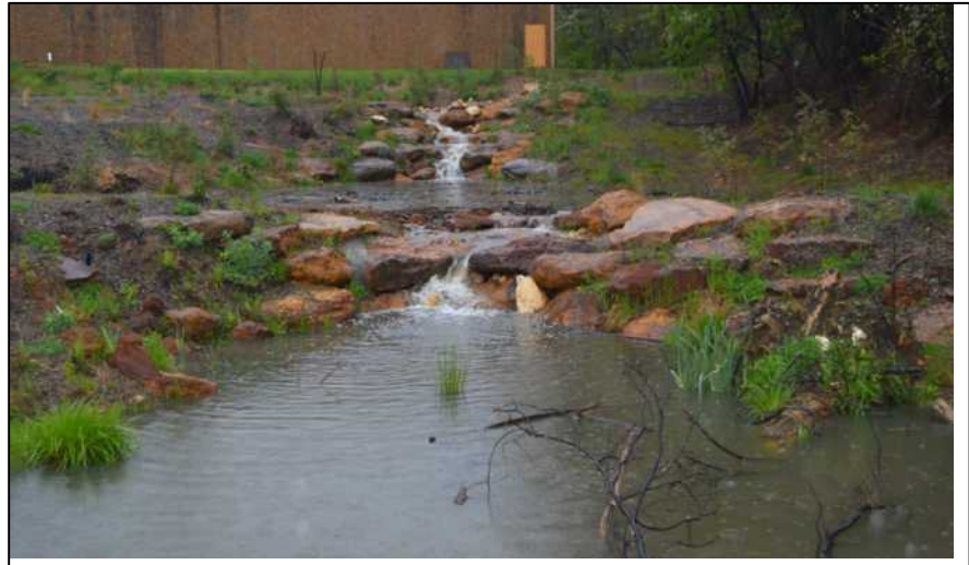
Figure 49. Gentle parabolic shape to keep flow from cutting around. Curved rack to widen flow. Flat placement of boulders to break flow. Tie in boulders extending into the berm and existing ground.
