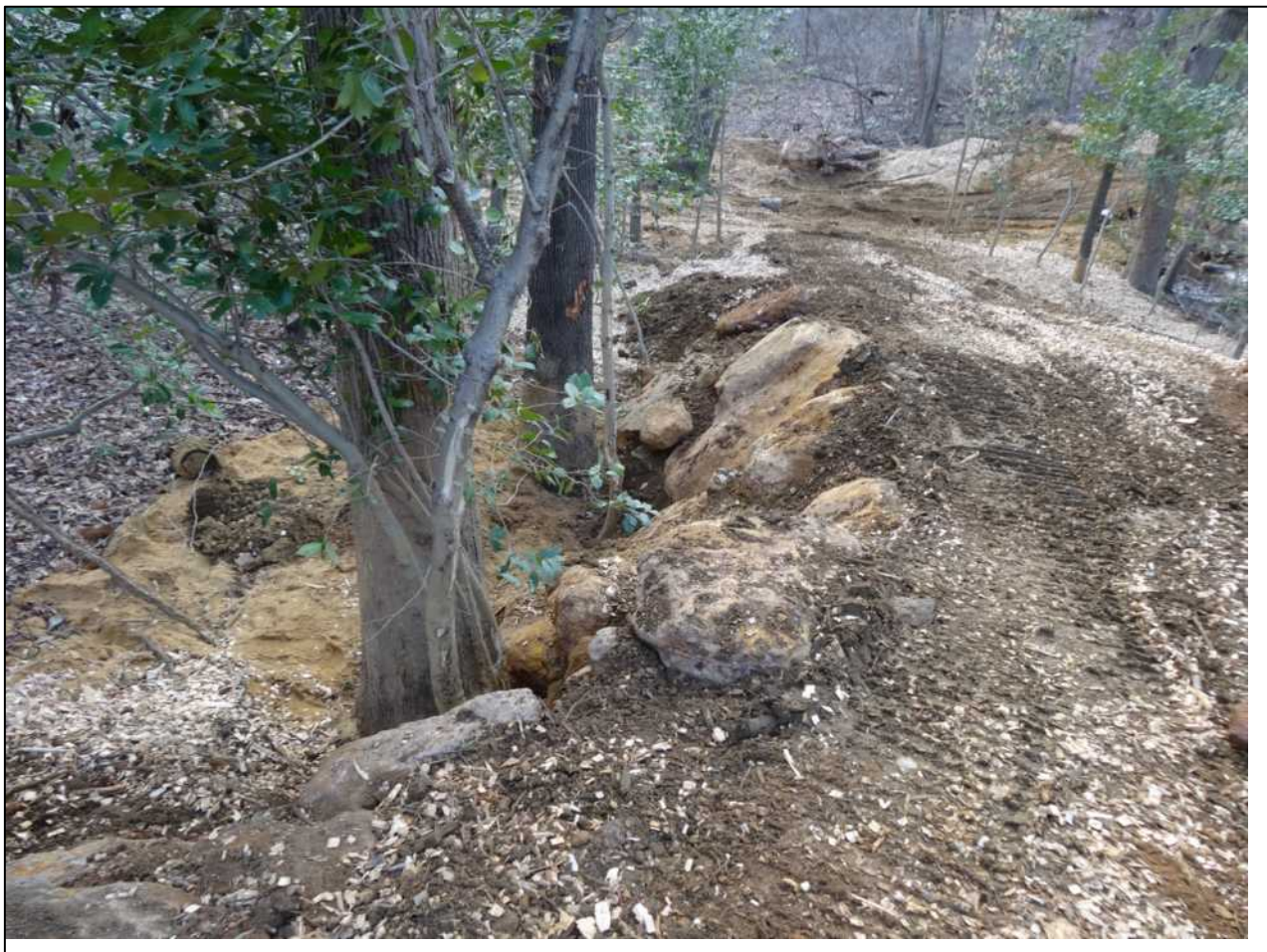
Figure 16. To avoid removal of trees that are close to the haul road, tree wells and boulder walls are available techniques. Rather than remove a tree that is on the edge of the haul road, keep the tree while ensuring that a tree well is created and maintained to avoid burying the trunk.
