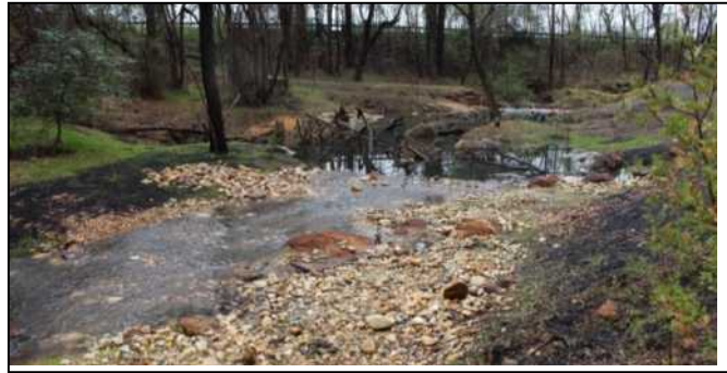
Figure 40. Riffle leading up to one-foot weir contains scattered erratic rocks that reduces energy by disrupting flow. Weir boulders are submerged under streamflow after storm event. Gentle parabolic shape of weir both spreads stream flow within the riffle and weir as well as prevents flow from cutting around the weir.
