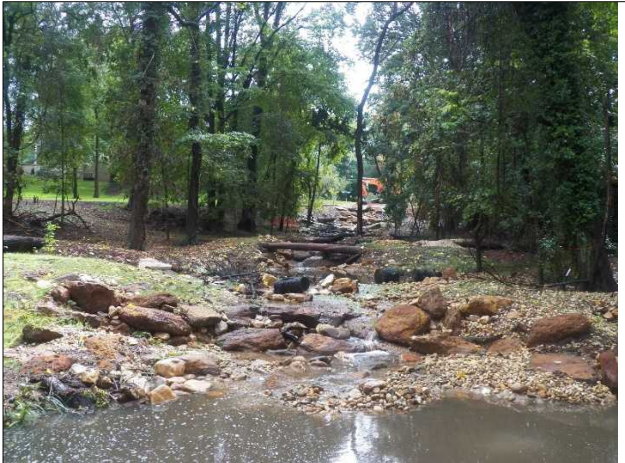
Figure 30. Weirs are placed to form a parabolic shape that is continued onto the bank. Footer boulders are submerged during wet period with downstream apron of river rock seen at water surface.
