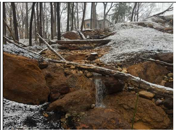
Figure 7. Example of a steep gully and exposed utilities restored with a step pool stormwater conveyance to capture stormwater (flowing down boulder) at the end of a dead end street and non-erosively convey and improve water quality before it enters a stream.
