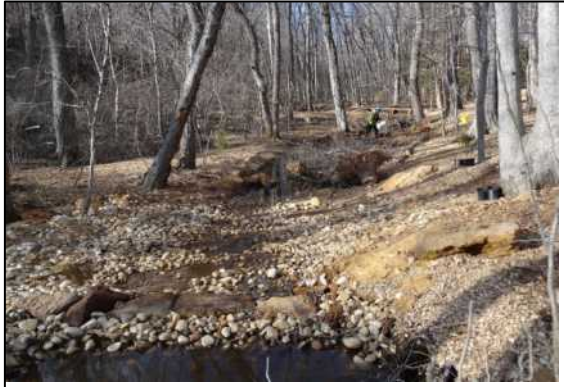
Figure 39. Riffle with scattered erratics extending upstream from weir boulders. Apron of river rock extends downstream from weir boulders and into the pool.
