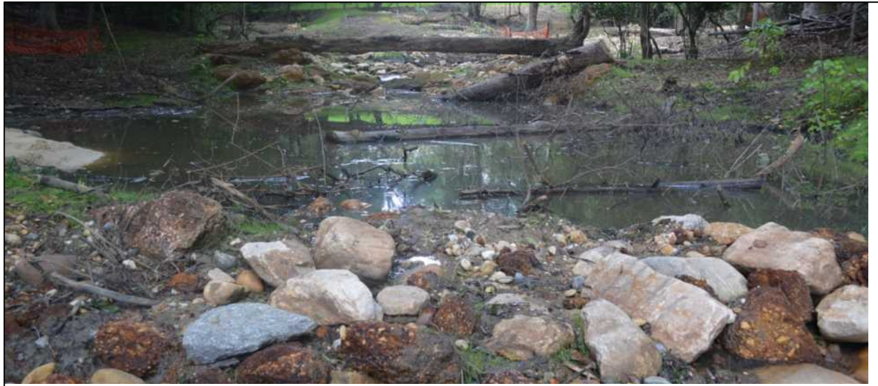
Figure 56. Abundant supply of woodchip, brush, branches and logs added to riffle-weirs, pools and riparian areas replenish some of the organic material lost to construction and help support multiple stream functions.
