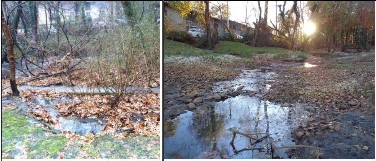
Figure 8. Example of just completed RSC restoration of a small stream near the mouth of a tidal river. Increased stormwater runoff from roads and parking lot eroded the wetland and stream complex, causing sediment to flow into the river.
